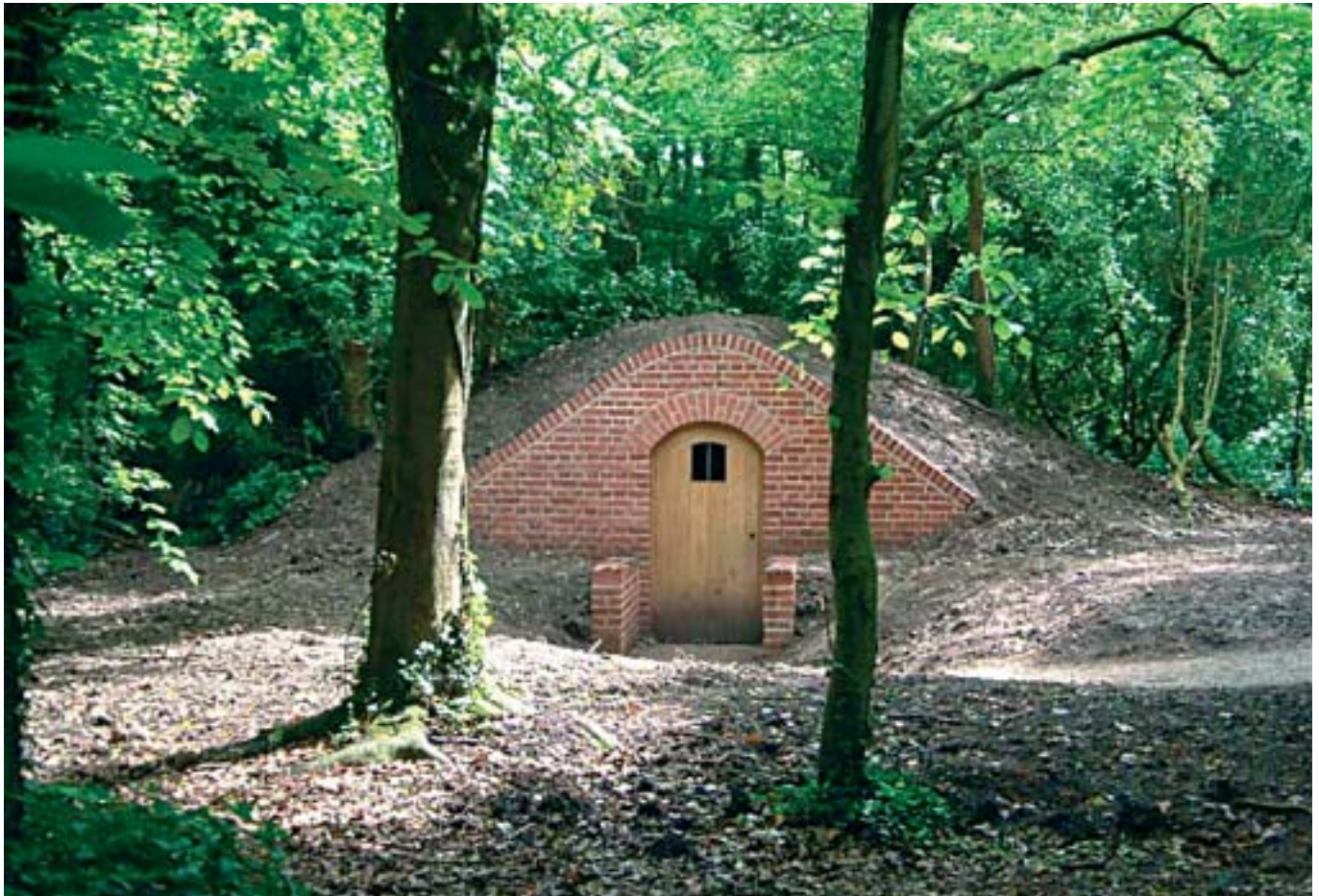
Work was completed on the Ice House in the spring of 2007
