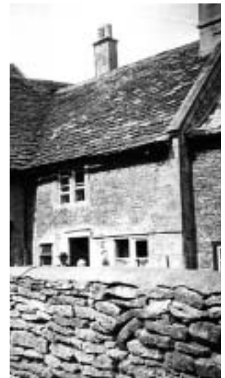
Adjoining buildings were demolished in the 1960s but knowledge of their existence helps to explain how the area was used in the past
