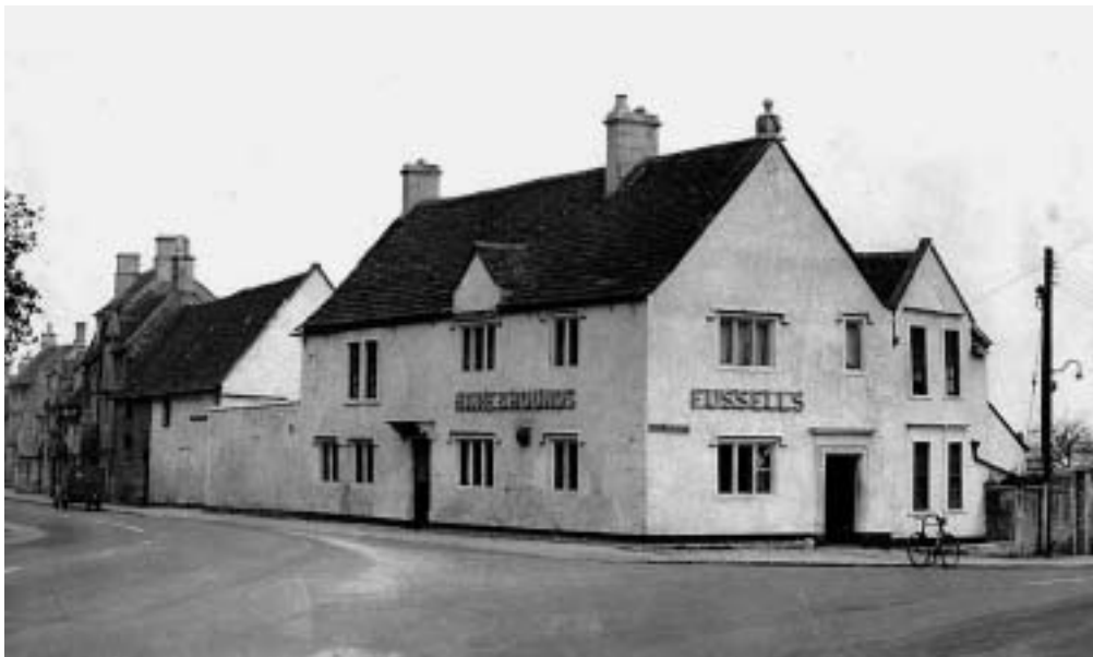
Historical photographs can provide valuable information. Here as seen in 1948 the original line of the gable of the Ostler's House provides justification for its rebuilding
