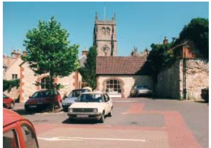
The 1930's shopfront restored as a link to the past use.
