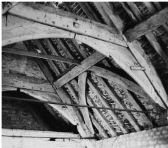
Roof of the Granary
