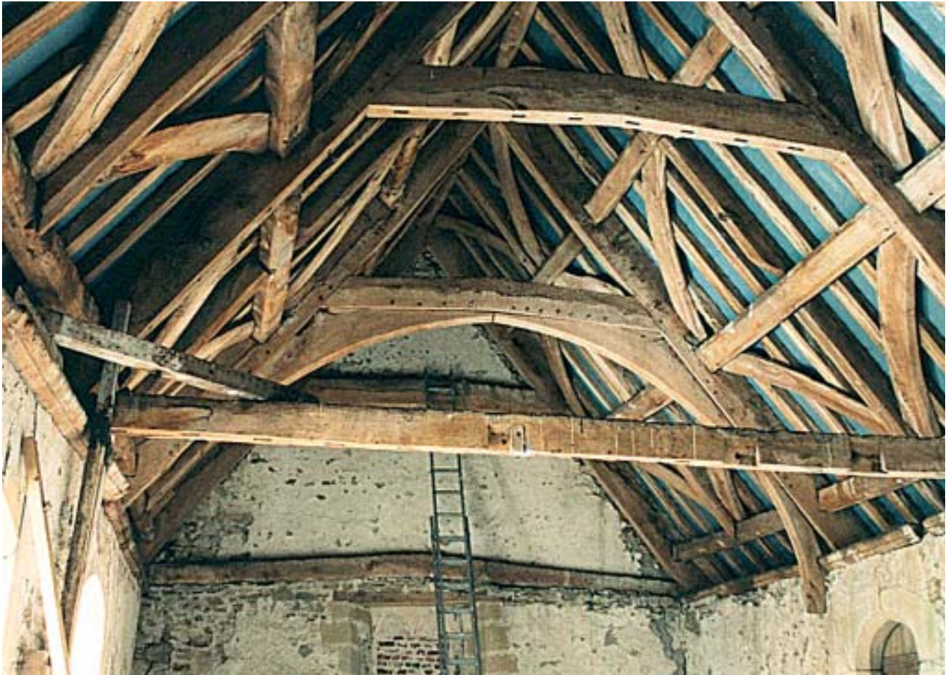
The first floor interior showing the main roof structure
