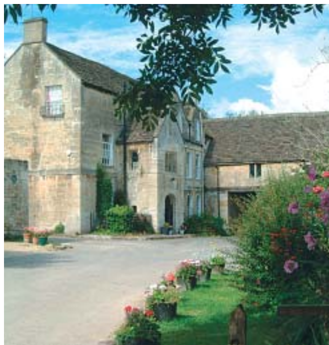
Roof of the Granary
