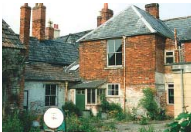
The rear of 21,23 and 25 Church Street following demolition of the factory buildings as seen in 1992.
