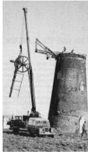
Removing the remains of the fantail staging 1969
