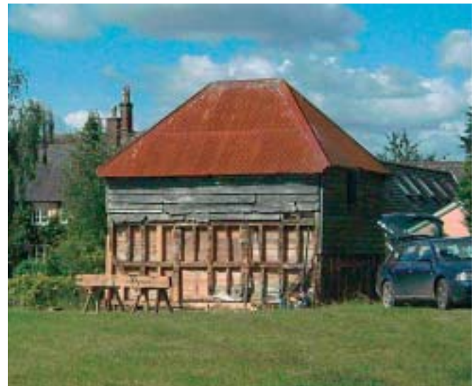
Work in progress in 2007 to repair the timber frame
