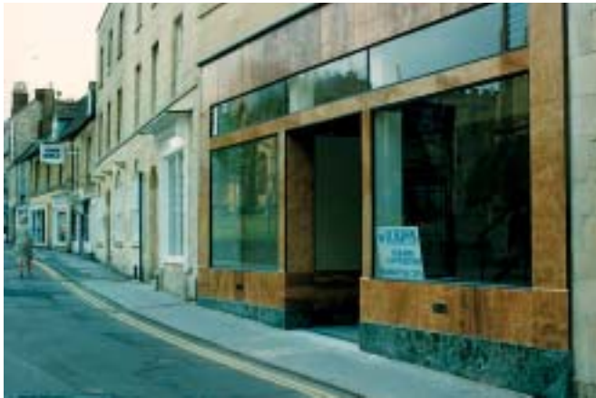
The 1930's shopfront restored as a link to the past use.
