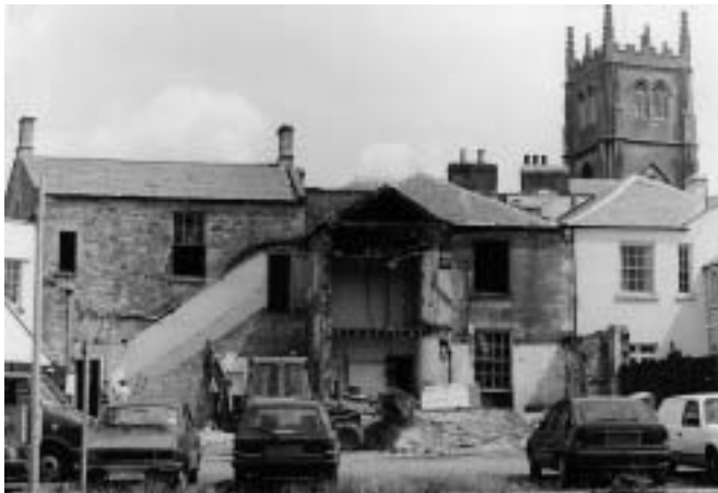
The rear of 13 and 15 Church Street as work started in 1989
