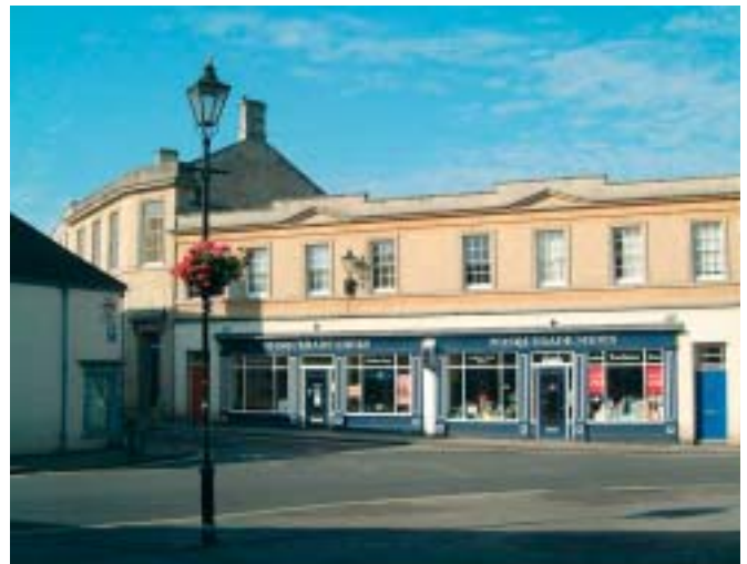
Church Street in 2007 is a very different place to that seen in the 1980s. All the shops are in use and the full potential of the buildings has been achieved and maintained.
